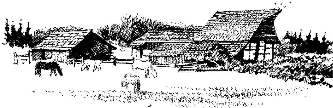
ABOVE. OLD BARN ON HAMMOND BAY ROAD.
